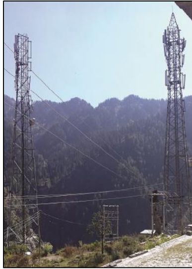
Image-2.6: Mobile Satellite Towers in Malana
